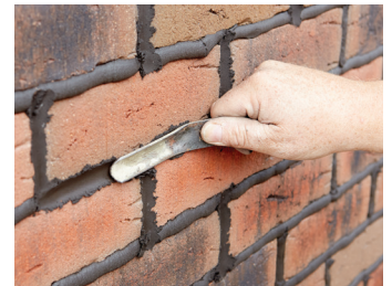
4. Mortar is tooled in the manner of traditional pointing.
