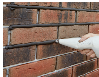
3. Specially formulated mortar is then piped into the brick joints.
