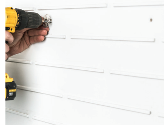
1. The ribbed backing panel is fixed to the substrate.
